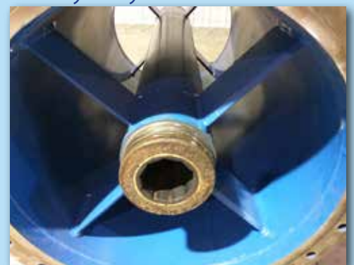
Plascoat ® PPA 571 Aqua provides excellent abrasion resistance. The above pipe carried potable water for one year and on inspection showed no sign of abrasion damage. Image courtesy of Diecron Inc., Macon, GA
