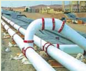
▼ Plascoat® PPA 571 lined pipes for desalination plants.
