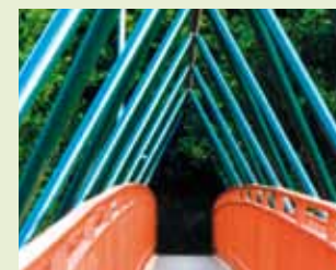
◀ Plascoat® PPA 571 in good condition after 20 years.
