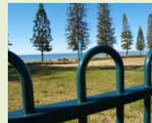
▼ The same fence re-coated in Plascoat® PPA 571 after 15 years.
