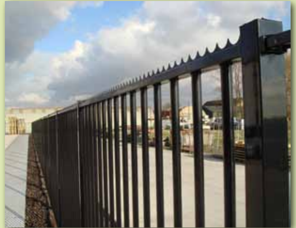
This ornamental perimeter fence is coated in Plascoat PPA 571
