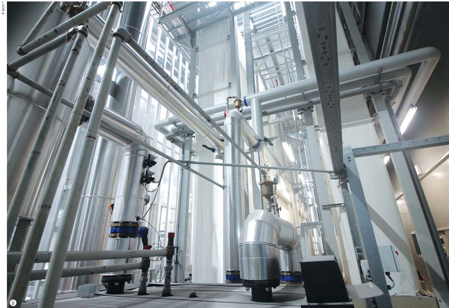
**Figure 8: The pre-treatment tunnel is divided into two parts: the initial steps and the alkaline etching process occur on one side, while the acid-based Oxsilan conversion steps are performed on the opposite side.**
